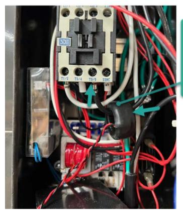
Step 4: Install the Current Transformer (CT)
