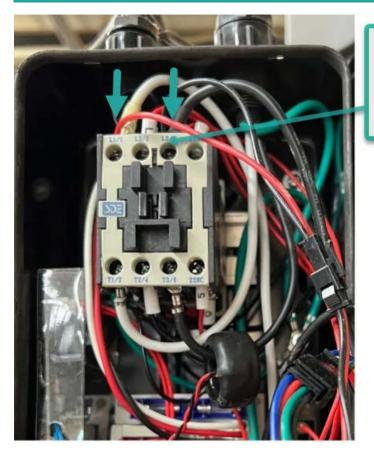
Step 3: Connect the AC Wires
