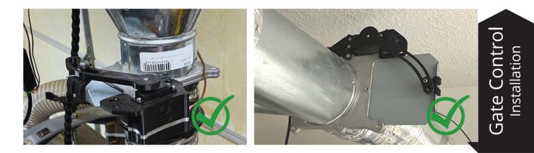
If the location of the existing blast gate does not allow for mounting the gate actuator as shown above, you can move the actuator to the other side of the blast gate by changing the direction of the Slide Bracket post.
